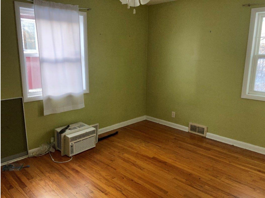
Attachment A: Pictures for 3457 Milwaukee Street
